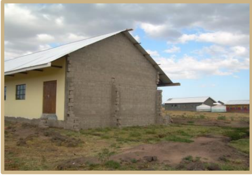
Meiorwa Dining Hall showing the extension
